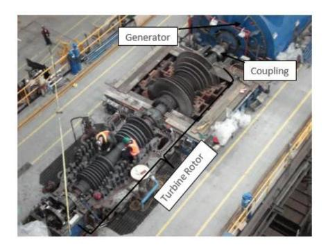
Figure 3: Turbine-Generator (with Turbine Casings Removed).
